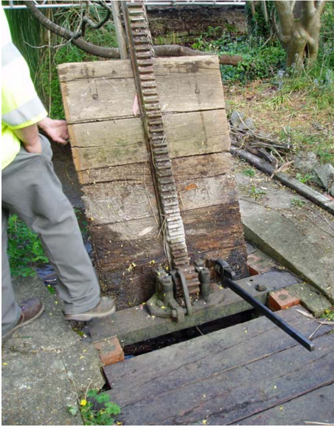
Photo 1 – Salmon Leap sluice hatch prior to refurbishment
