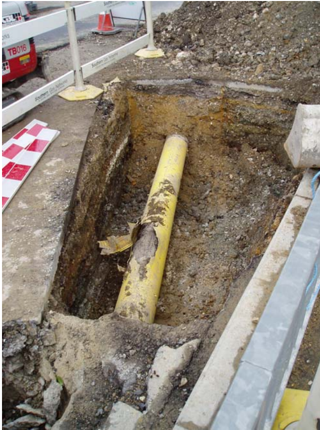
Photo 2 – Excavation of the gas networks (The Borough)
