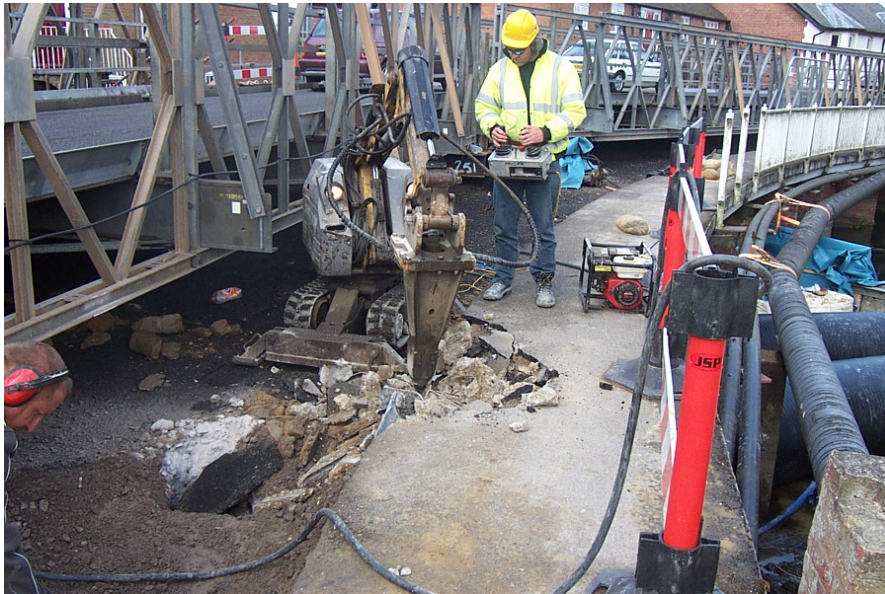
Photo 5 – Commencement of the demolition works
