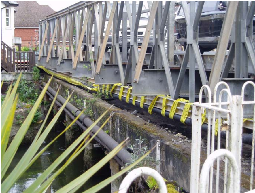
Photo 3 – Diversion of the electrical services beneath the temporary bridges
