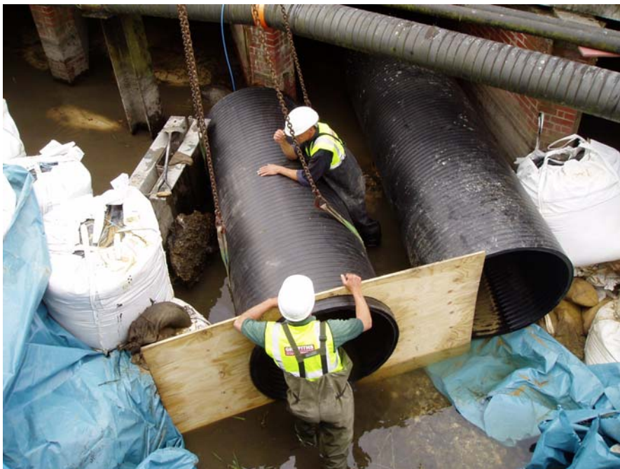
Photo 4 – Installation of the additional pipes through the dams
