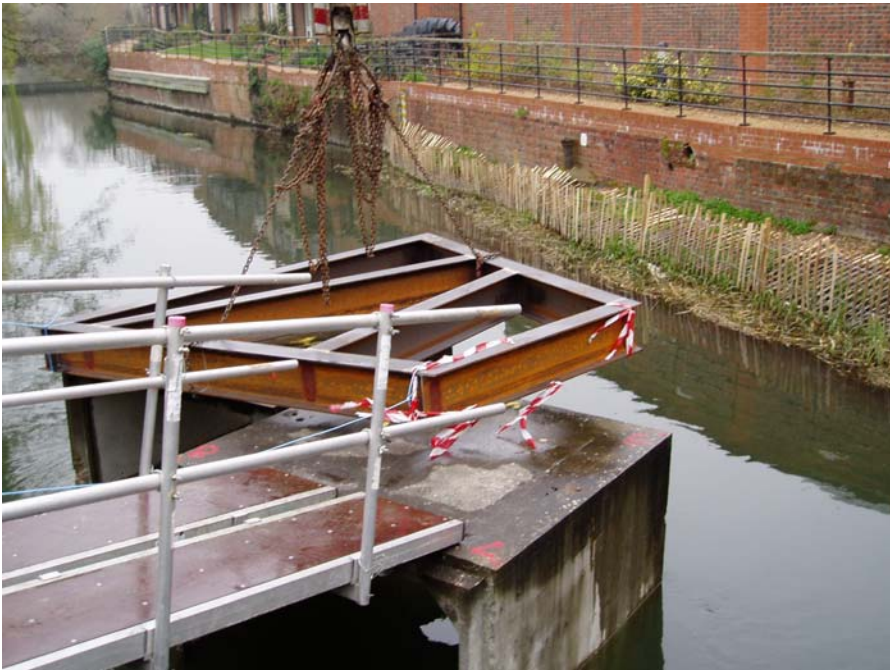
Photo 2 – Temporary footbridge centre pier capping piece installation
