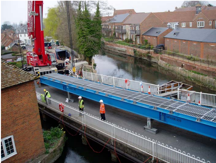
Photo 4 – Temporary footbridge erection (pre-lift)
