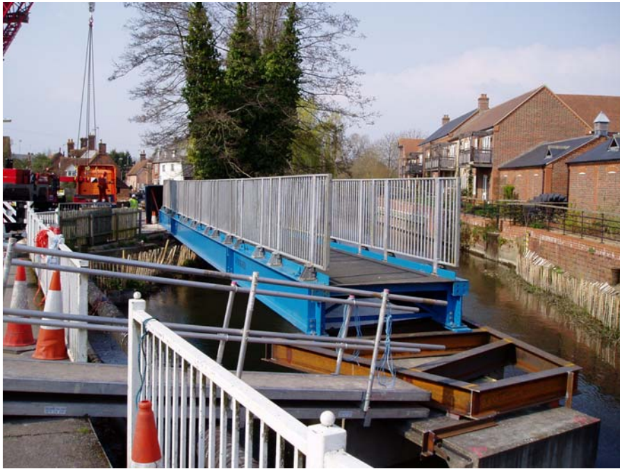
Photo 6 – Temporary footbridge first section
