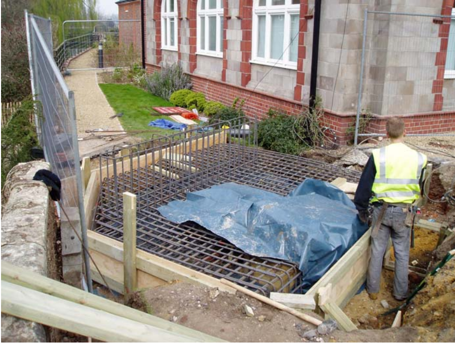
Photo 1 – Temporary footbridge foundation construction (Old Tannery end)
