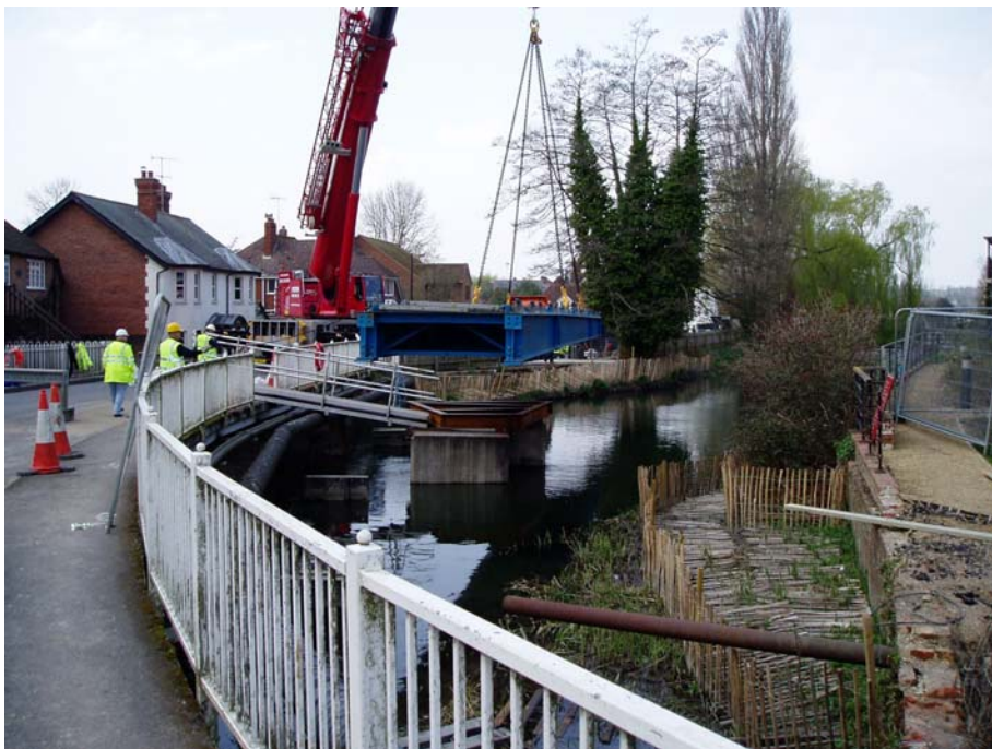
Photo 5 – Temporary footbridge erection (during lift)
