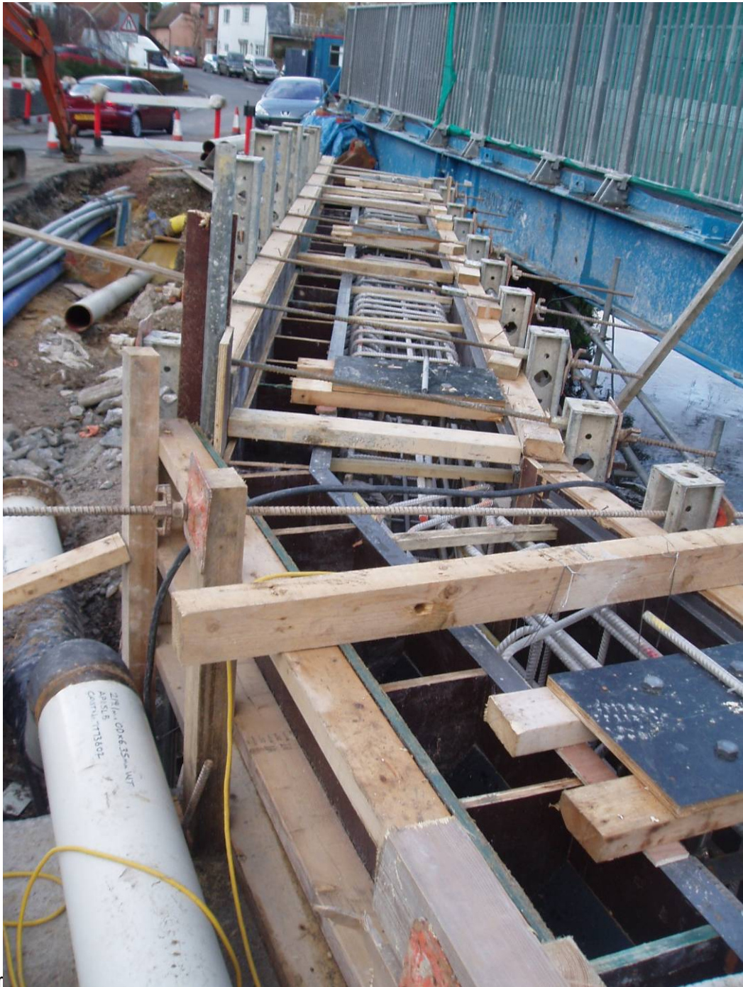
Photograph 4 Northern edge beam
