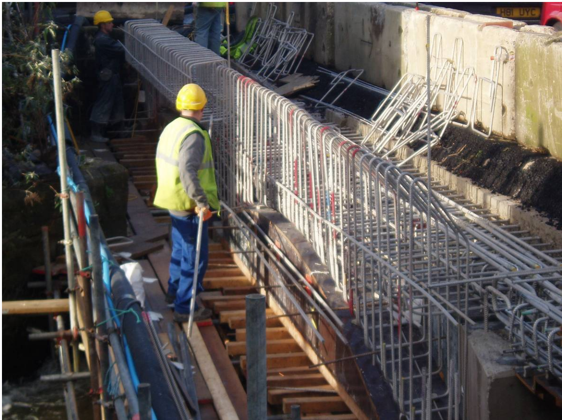
Photograph 2 Span 3 Preparation works in progress
