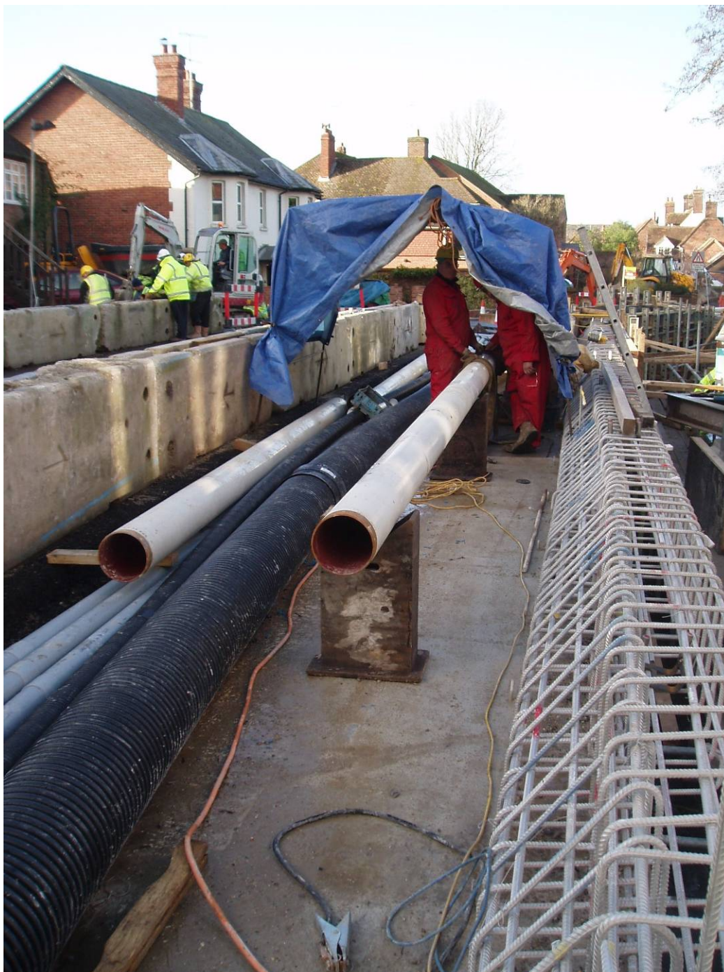
Photograph 1 Gas duct welding in progress
