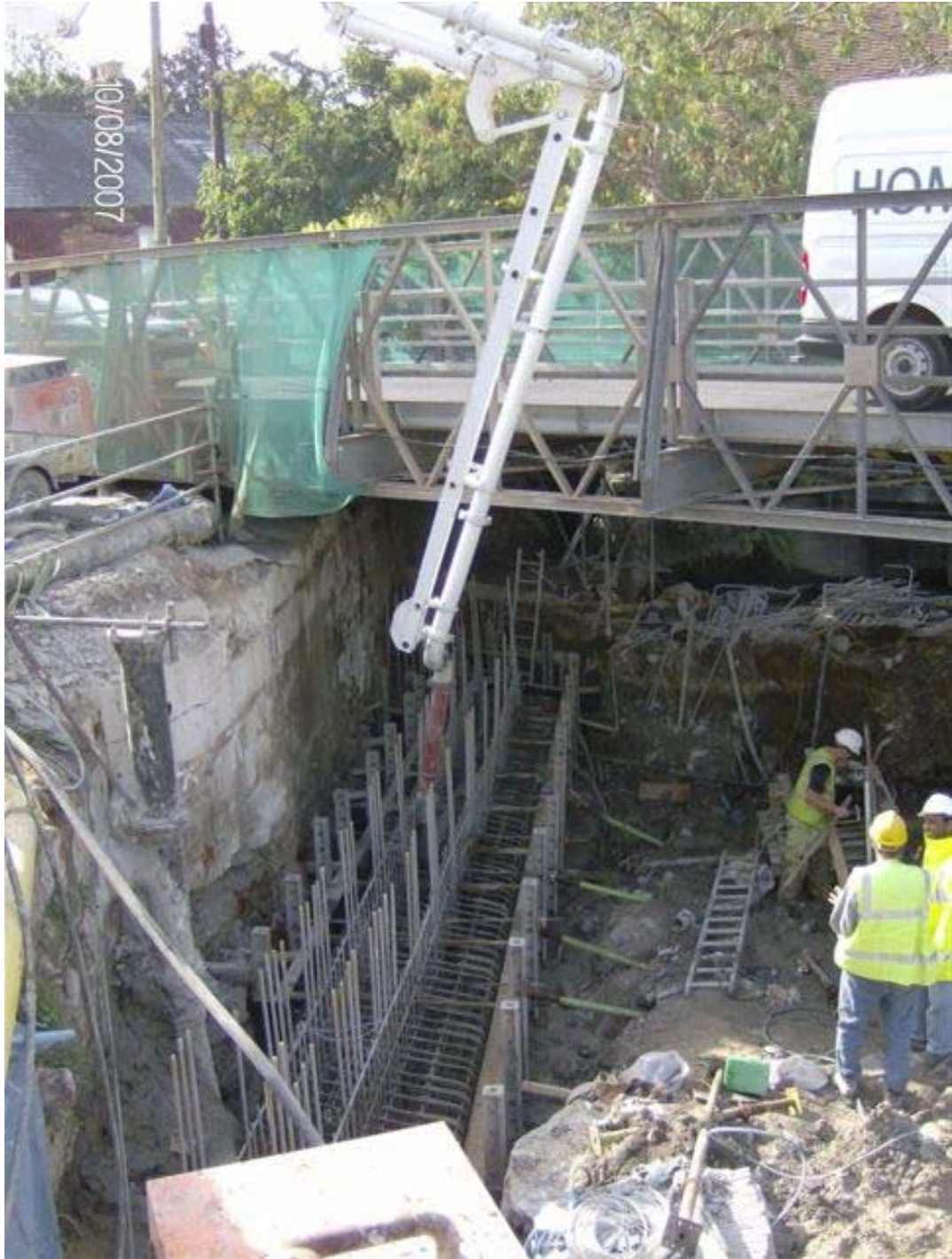
Photograph 3 The Eastern Abutment Pile Cap in Span1
