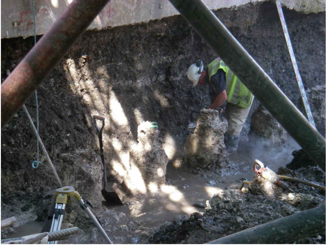
Photograph 1 Exposing the pile caps in Span 1
