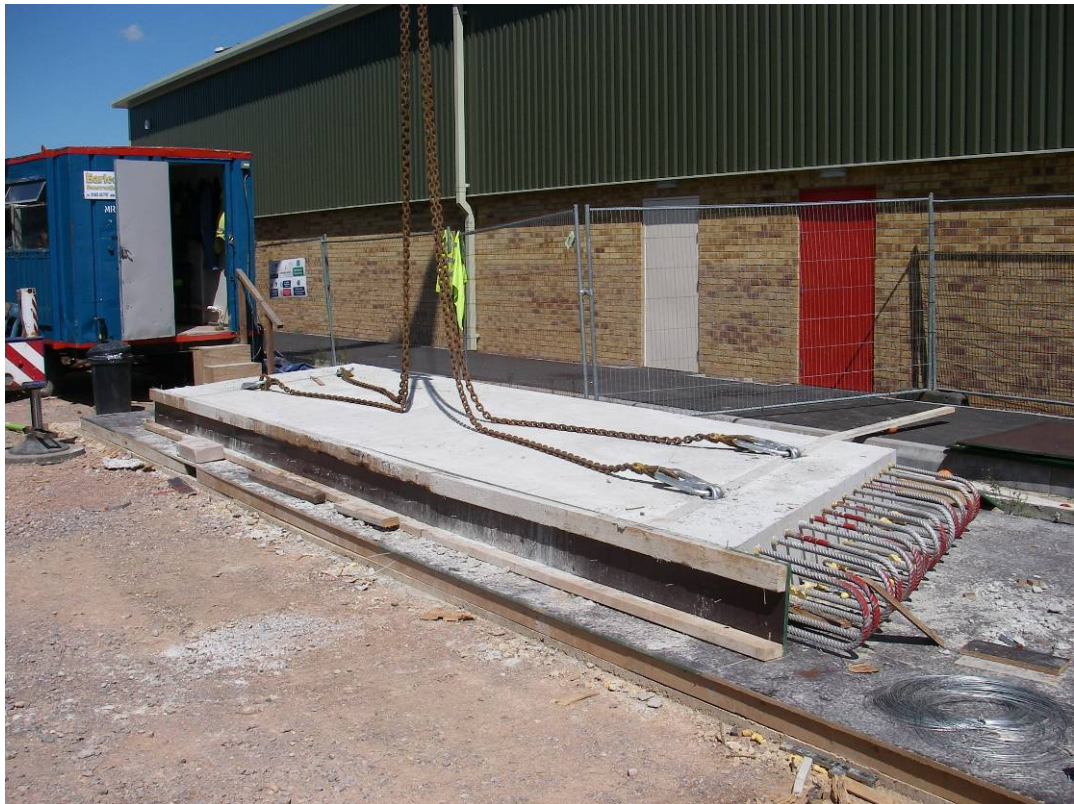
Photograph 2 Lifting the Bridge Deck Units, on the Downton Industrial Estate
