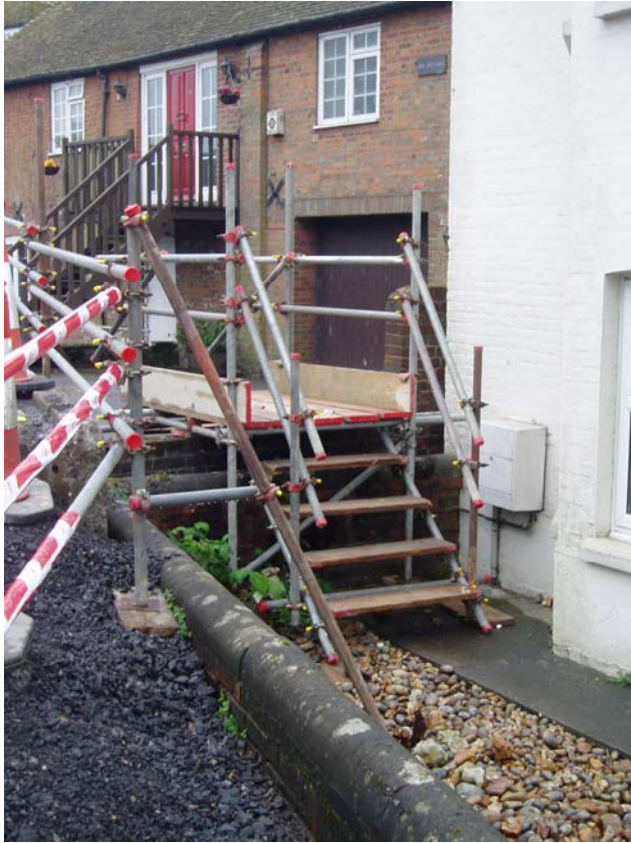
Photo 1 – Temporary pedestrian access to The Old Mill
