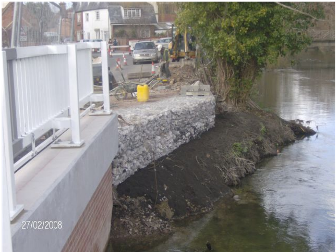
The Reinstated Western Footway Approach
