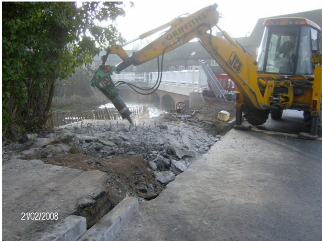
Breaking Out the Western Foundation To The Temporary Footbridge
