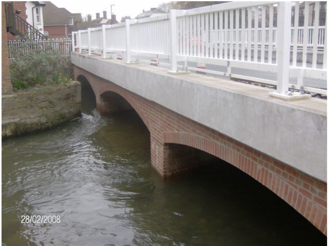
Photograph 1 The Southern Façade From Waterside Mill
