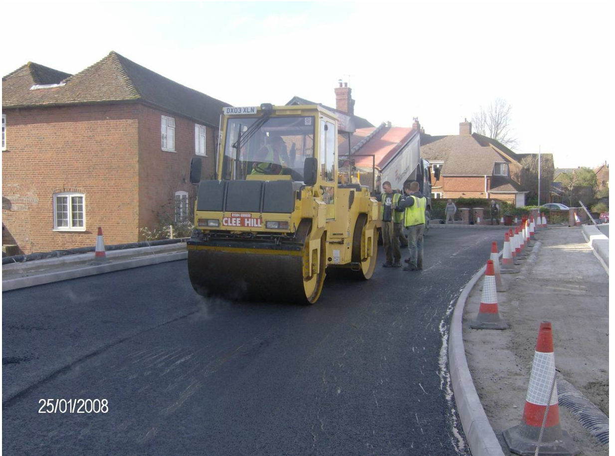
Resurfacing The New Bridge Deck
