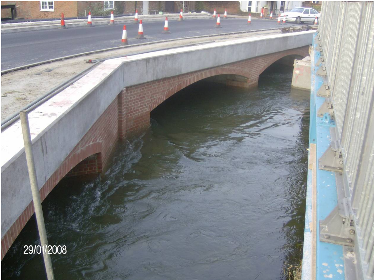
Photograph 1 The Northern Façade
