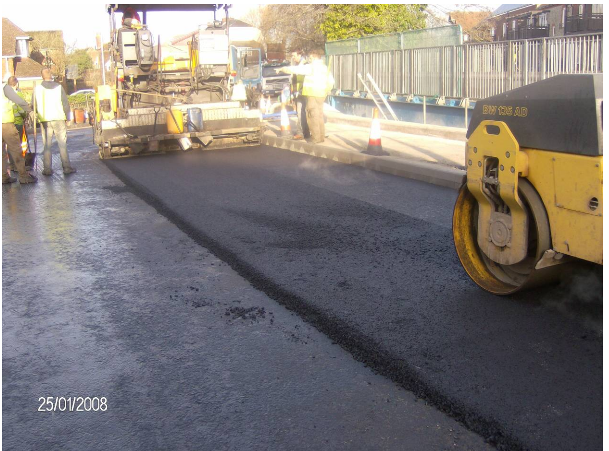
Resurfacing the New Bridge
