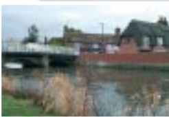
▲ Flood walls alongside the River Avon, downstream of the Iron Bridge
